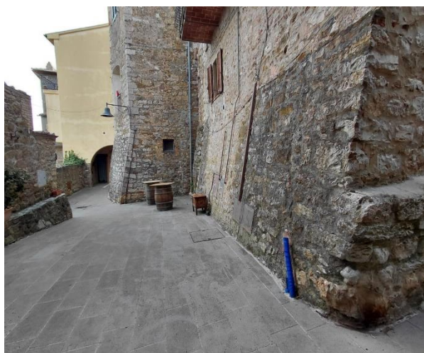
13 continuation along via Solferino
