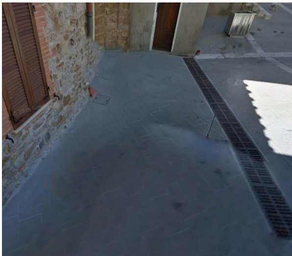
19 ramp, beginning of Via Solferino from Piazza Mario Signori
